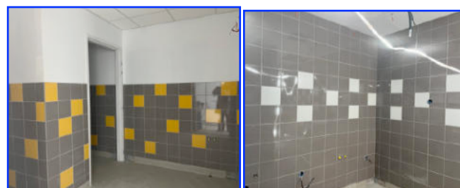
Carrelage, faïence, entreprise Veyron
